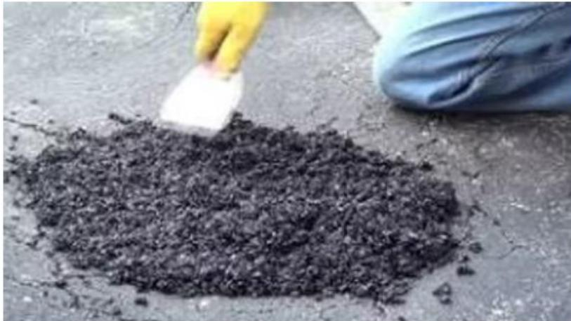
Potholes are holes in the roadway that vary in size and shape. A pot hole is a structural failure in a road surface. Hitting a pothole can not only cause damage to a vehicle's shocks and suspension, it can also cause the driver to lose control of his or her vehicle.
